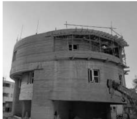
World's largest 3D printed complex in final stages of completion for BRO Ladakh Air Despatch establishment at Chandigarh, Source: BRO images
