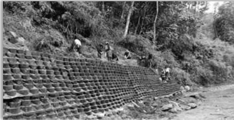
Geo Breast Wall on Sangklang-Toong Road in Sikkim, Source: BRO images
