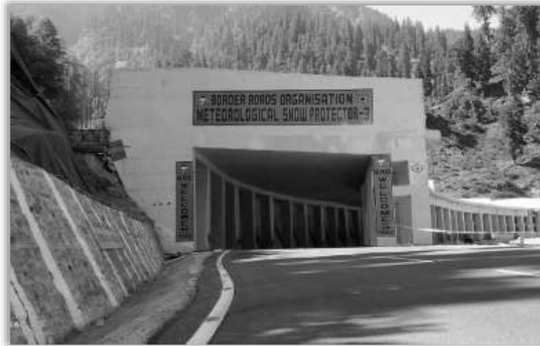
Snow Gallery near South Portal of Atal Tunnel, Source: BRO images
