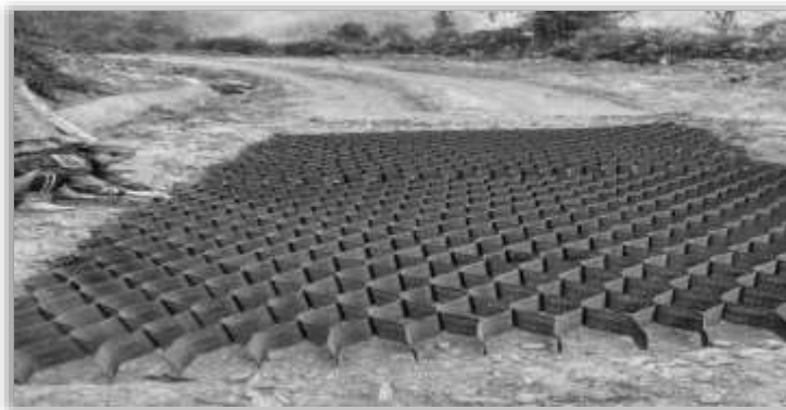
Hapoli-Sarli-Huri Road in Arunachal Pradesh, Source: BRO images
