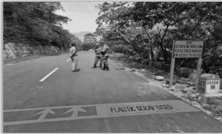
Resurfacing using plastic waste onBalipara-Charduar-Tawang Road, Source: BRO images
