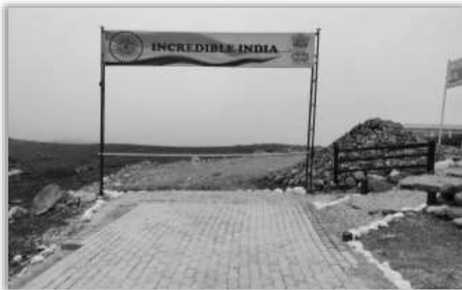
ILCB Pavement on Bumla-Bumla PP Road, Source: BRO images
