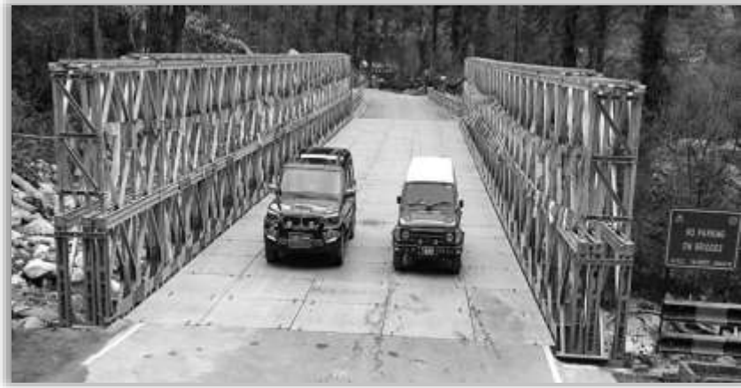
CL-70 Double Lane Modular Bridge on Flag Hill-Dokala Road in Sikkim, Source: BRO images
