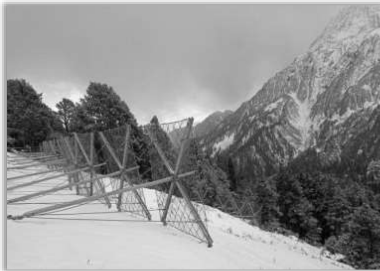
Snow Erodox System at South Portal of Atal Tunnel, Source: BRO images
