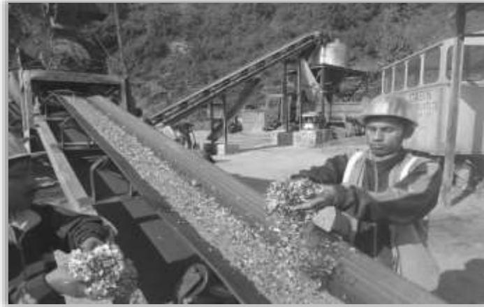
Mixing of dry plastic waste with aggregate, Source: BRO images
