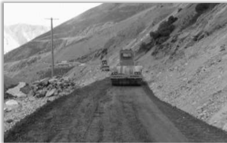
Sumna-Rimkhim Road in Uttarakhand, Source: BRO images
