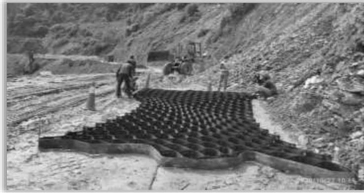
Balipara-Charduar-Tawang Road in Arunachal Pradesh, Source: BRO images
