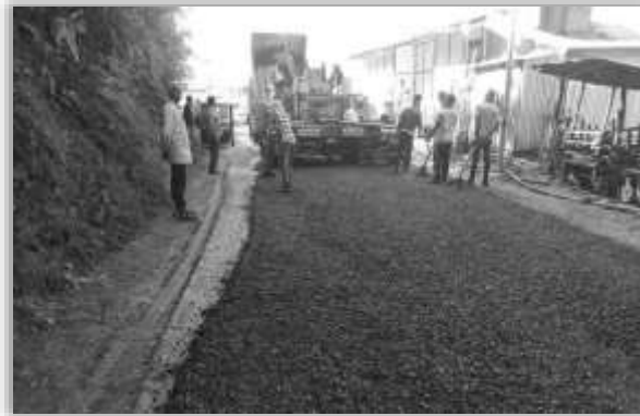
Resurfacing using plastic waste on Hnathial-Sangau-Saiha Road in Mizoram, Source: BRO images
