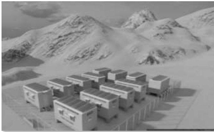
Carbon Neutral Habitat at Hanle (15000 feet), Source: BRO images
