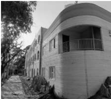
World's largest 3D printed complex in final stages of completion for BRO Ladakh Air Despatch establishment at Chandigarh, Source: BRO images
