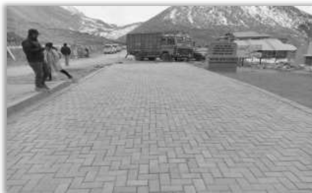
ILCB Pavement at Changla Pass on Karu-Tangtse Road, Source: BRO images
