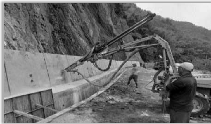
Pre-cast Breast Wall & Drain on Along-Yingkiong Road, Source: BRO images
