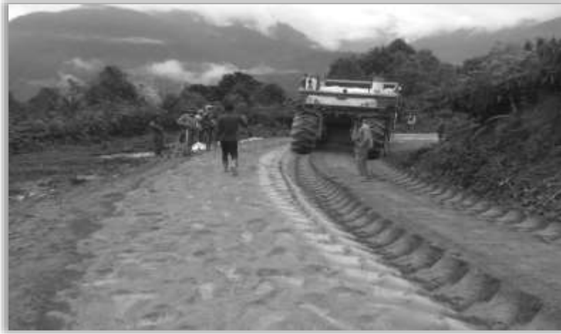
Hapoli-Sarli-Huri Road in Arunachal Pradesh, Source: BRO images
