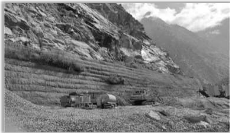
Rockfall Embankment on Joshimath-Mana Road, Source: BRO images
