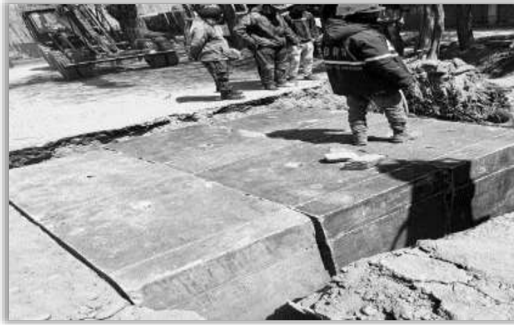
Construction of Precast Box Culvert in Ladakh, Source: BRO images
