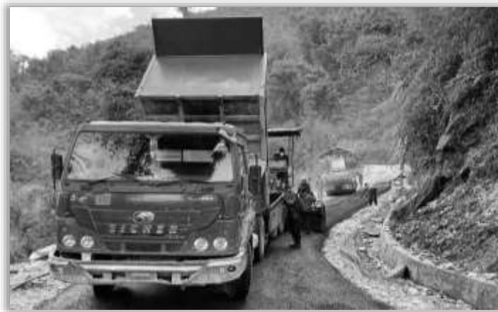
Black Topping using plastic waste on Hapoli-Sarli-Huri Road, Source: BRO images
