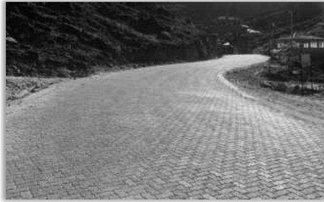
ILCB Pavement on Balipara-Charduar-Tawang Road (Sela Top) , Source: BRO images
