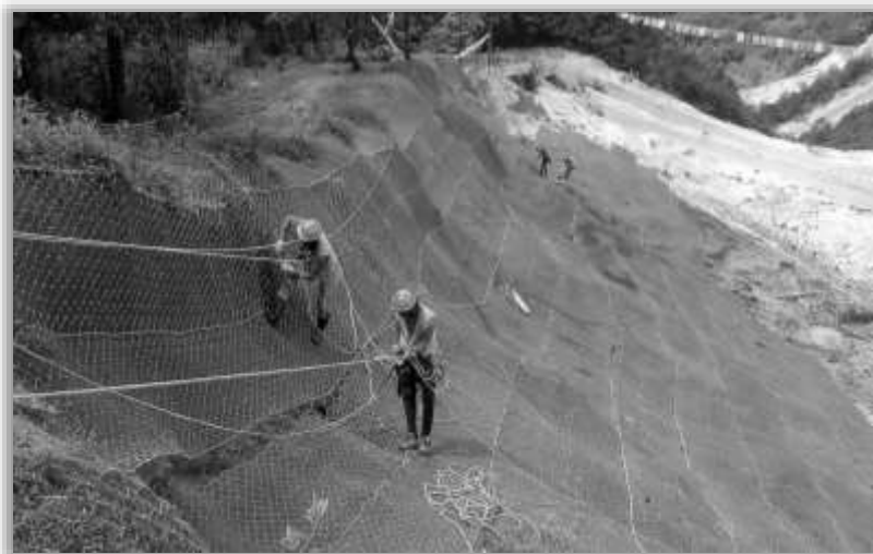
Geo Synthetics on Balipara-Charduar-Tawang Road, Source: BRO images
