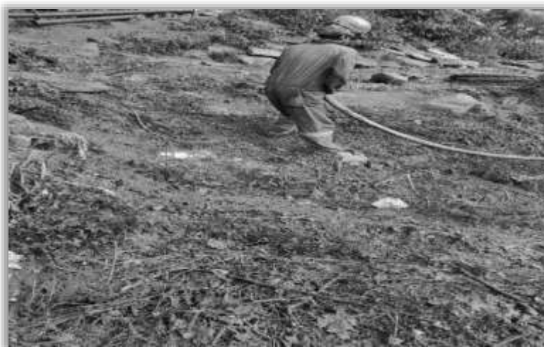
Hydro Seeding on approach to South Portal of Atal Tunnel, Source: BRO images
