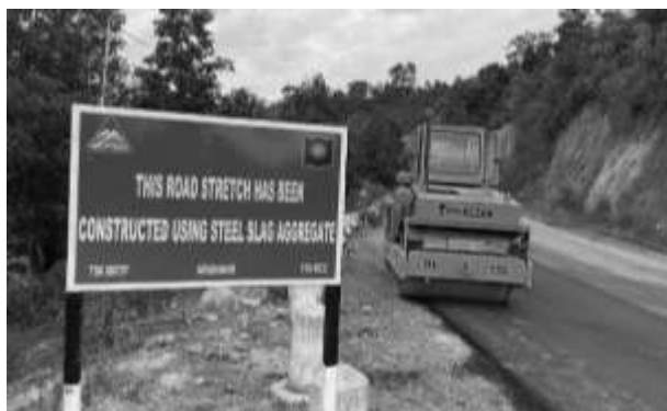
Road Stretch of Joram-Koloriang Road constructed using Steel Slag, Source: BRO images
