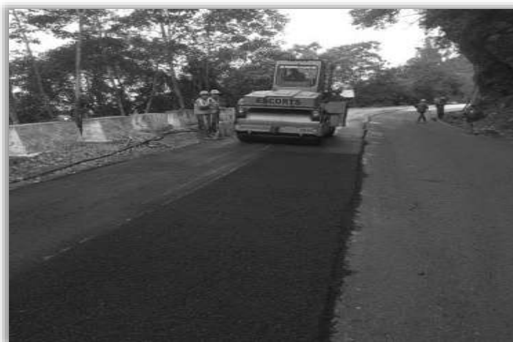
Resurfacing using plastic waste on Phuentsholing–Thimphu Road in Bhutan, Source: BRO images
