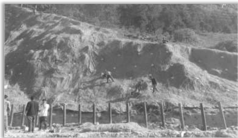
Secured Drapery with Micro Piling Work on Joshimath-Mana Road, Source: BRO images
