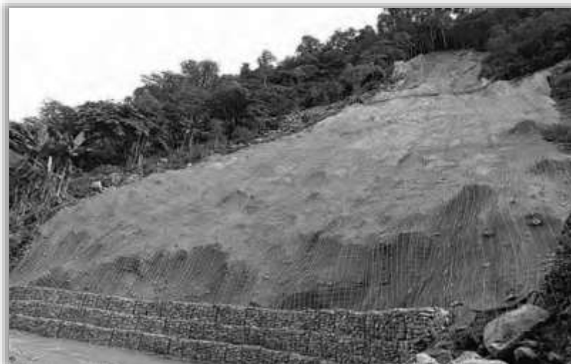
Biodegradable Coir reinforced with Gabion Wall on TCC-Maza Road, Source: BRO images
