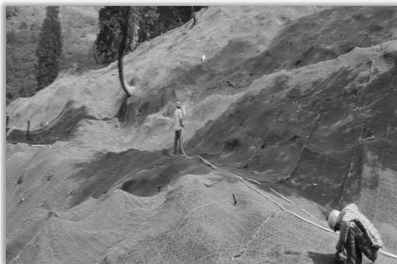
Reinforced Geomat on approach to South Portal of Atal Tunnel, Source: BRO images
