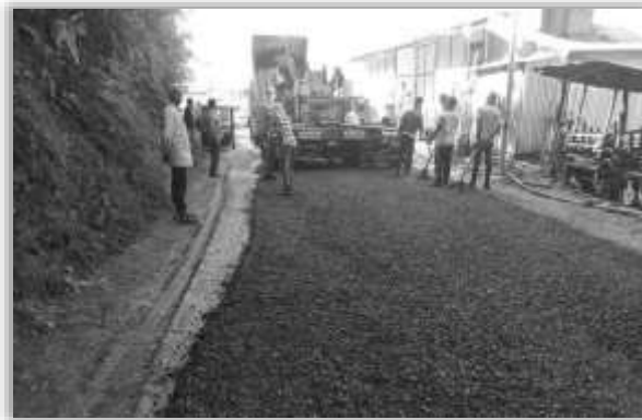
Resurfacing using plastic waste on Hnathial-Sangau-Saiha Road in Mizoram, Source: BRO images
