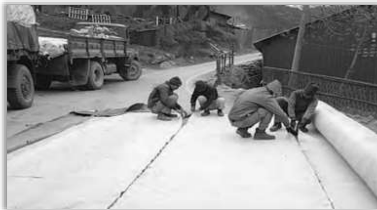
GCCM being prepared to make drains along road TCC- Taksing, Source: BRO images
