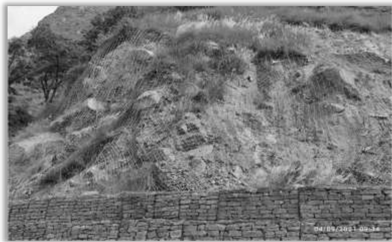
Drapery with Hill Side Gabion Wall on Joshimath-Mana Road in Uttarakhand, Source: BRO images
