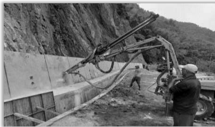
Pre-cast Breast Wall & Drain on Along-Yingkiong Road, Source: BRO images
