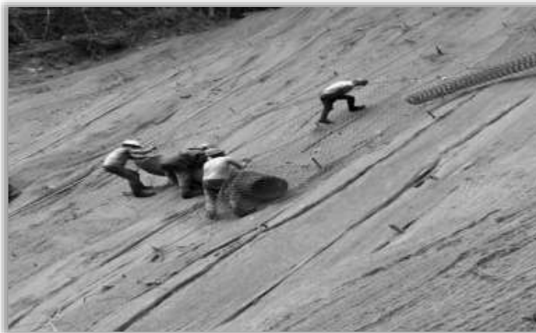
Geo Synthetics on TCC-Taksing Road, Source: BRO images
