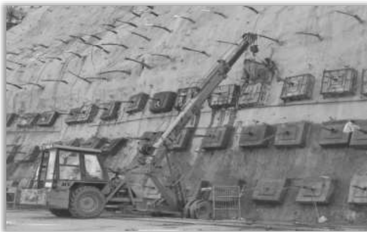
Pre-Stressed Cable Anchor on approach to South Portal of Atal Tunnel, Source: BRO images
