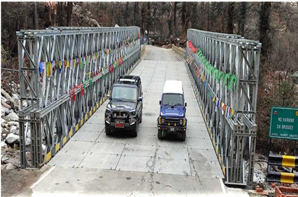
Class 70 Double Lane Modular Bridge at Flag Hill
